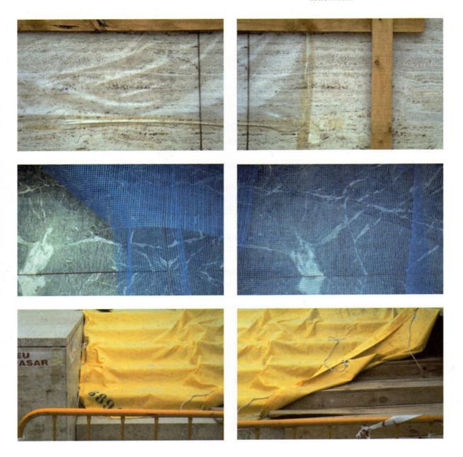
Figs. 13/14: Wooden frame on Roman travertine. Figs. 15/16: Blue plastic mesh on alpine marble. Figs. 17/18: Yellow tarp on travertine stairs.
