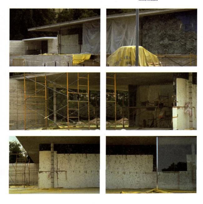
Figs. 1/2: Restoration of a reconstruction. Figs. 3/4: Steel scaffold below roof plane. Figs. 5/6: Styrofoam on alpine marble.
