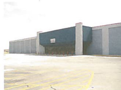
Empty Wal-Mart Supercenter, Beaver Dam, Wisconsin (Photograph by Wilbur E. Selbrede)
